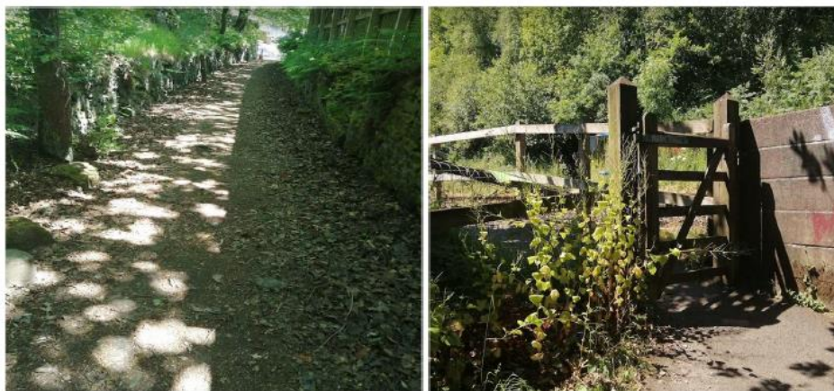
View of approach (looking towards Moorgate St, and pedestrian gate at railway boundary)
