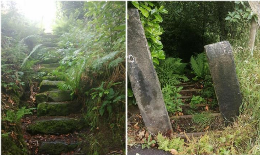
View looking up to Ladcastle Road and down the steps from Ladcastle Rd
