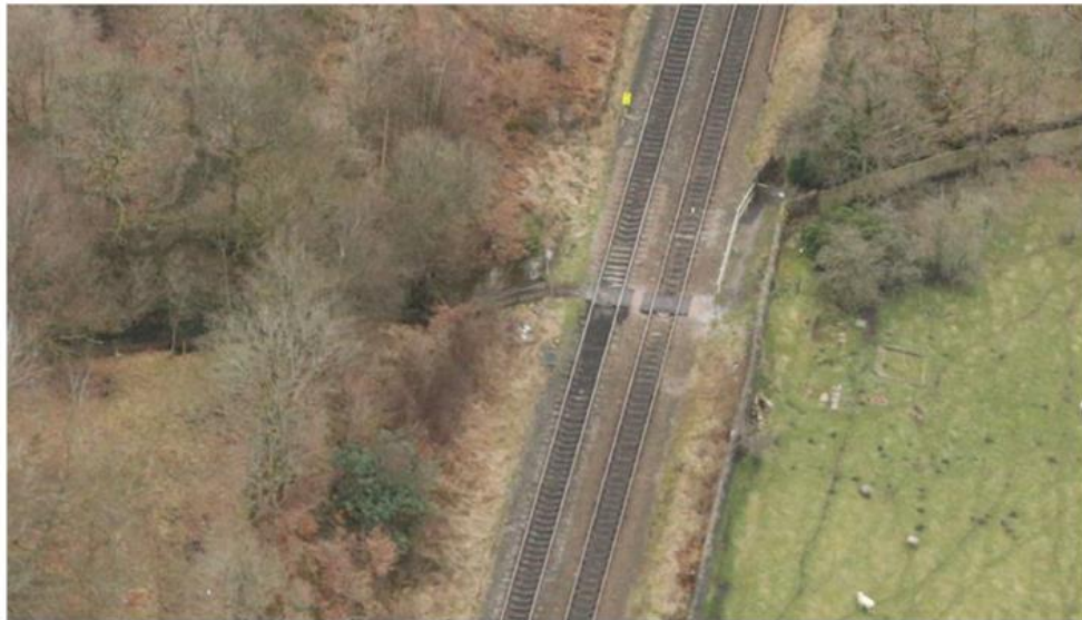
Ariel view of Moorgate Halt LC
